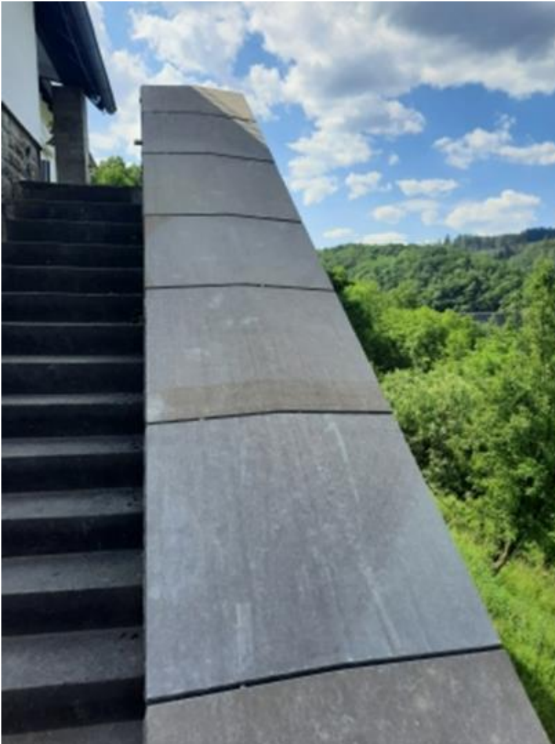
A successful renovation of the historic building ( Link to high-resolution photo)
