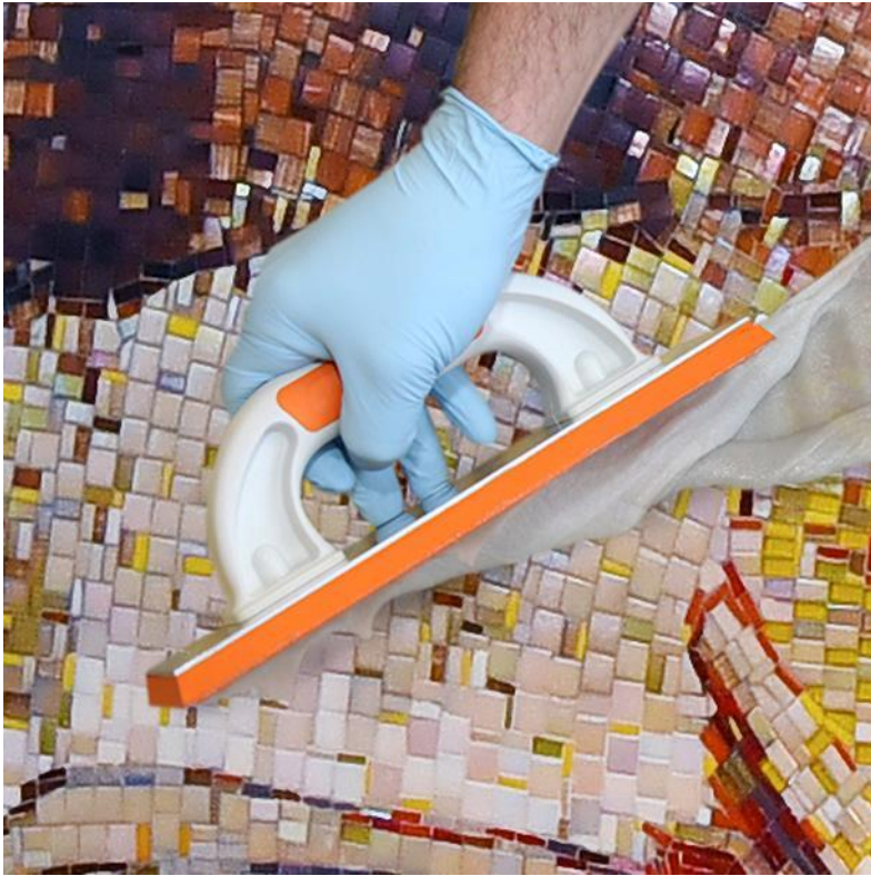
Jointing with PCI Durapox Premium Harmony ( Link to high-resolution photo )
