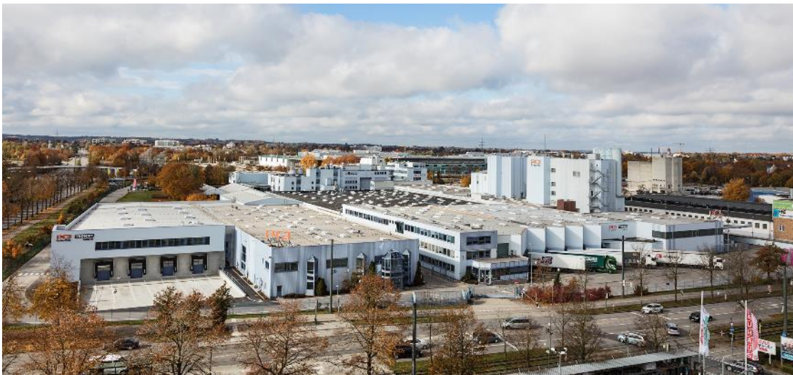
PCI-Headquarters in Augsburg ( Link to high-resolution photo )
