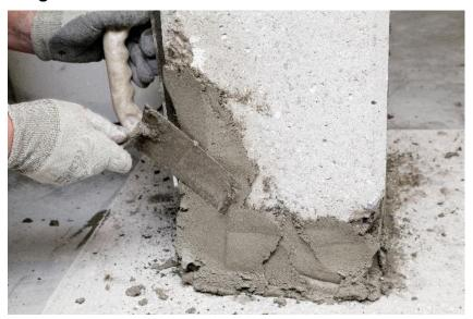
PCI system for concrete repair with static requirements (e.g. columns, balconies and stairs)) (©PCI Augsburg GmbH, Link to high-resolution photo).
